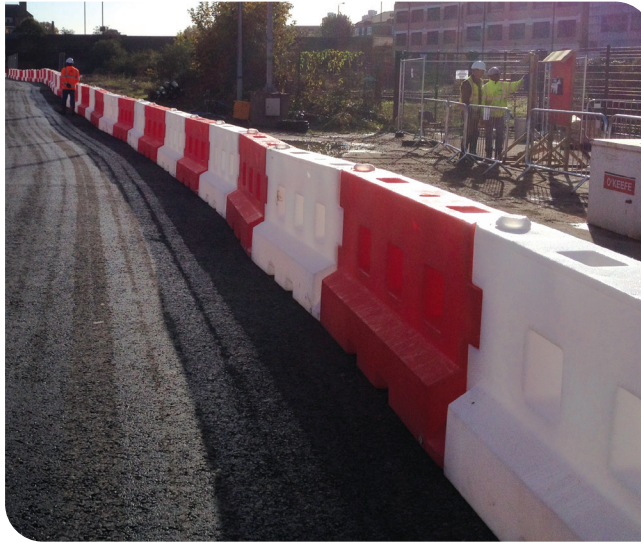
GB2's forming road perimeter on site
