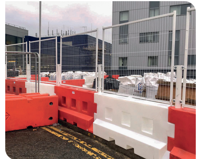
GB2's on site with mesh fence
